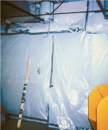
Photo 8: Full containment on large job
